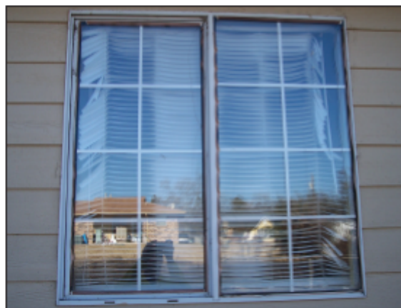
Radiant heat melted the interior blinds.
