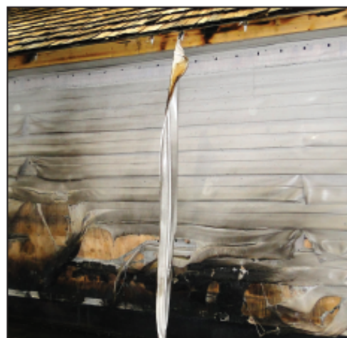
This vinyl gutter melted from heat, exposing the wood and roof edge to embers and direct flame. Photo by Institute for Business and Safety Research Center.
