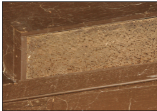
This screen prevented embers from entering. Photo by Institute for Business and Safety Research Center.
