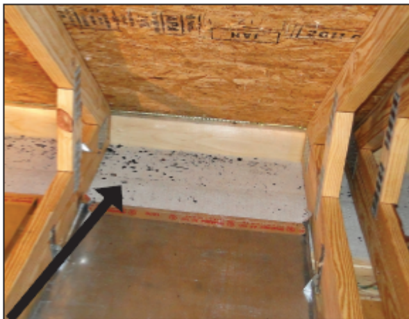
Without roof edge flashing, embers can enter into the attic. Photo by Institute for Business and Safety Research Center.
