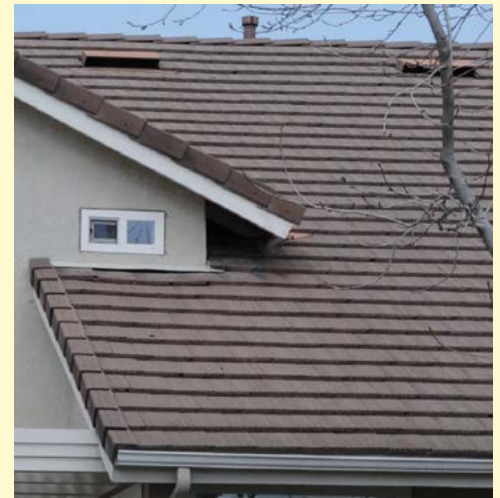
Use ignition-resistant, Class A-rated roofing materials and keep roof surfaces clear of debris.
