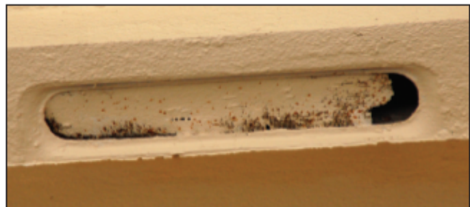
Vents can clog. This vent was painted over, reducing its effectiveness in providing ventilation. Photo by Institute for Business and Safety Research Center.
