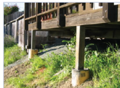
Use noncombustible materials when building a deck. Never store flammable materials on top of or beneath the deck.
