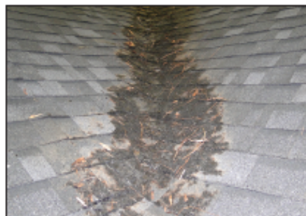
The pine needles on this roof burned, but the Class A roof did not. Photo by Institute for Business and Safety Research Center.
