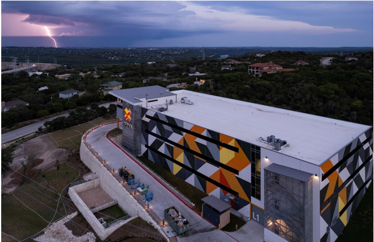
X-Space Luxury Garage Condos – Ranch Road 620 & Cloudy Ridge
